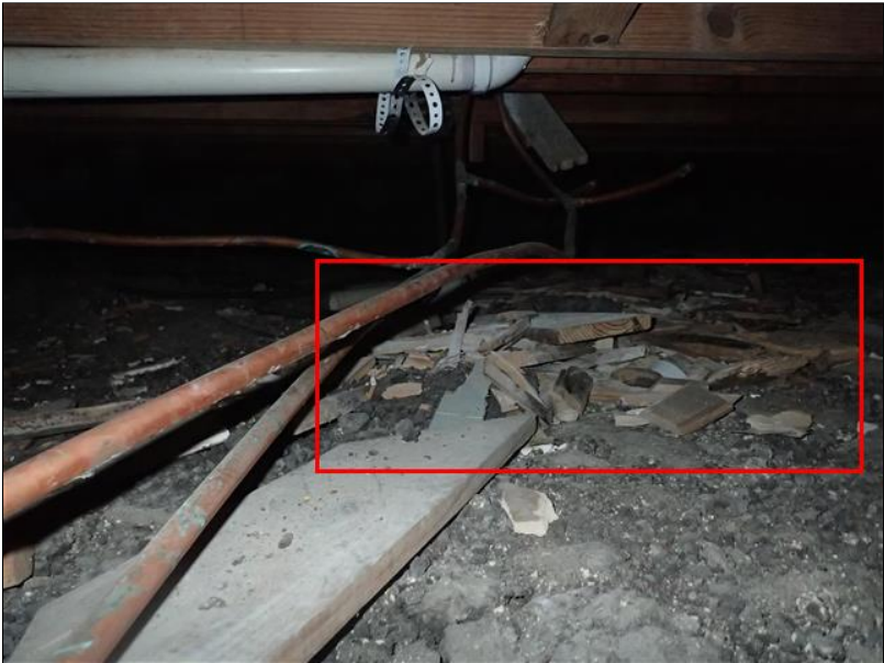
A. Item 1(Picture) Crawl space debris
