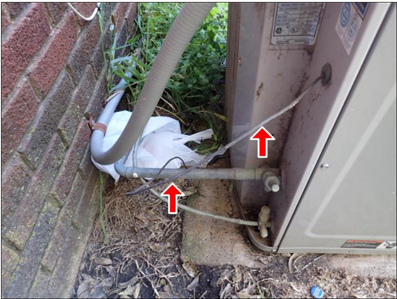
B. Item 8(Picture) A/C thermostat wire, north side
