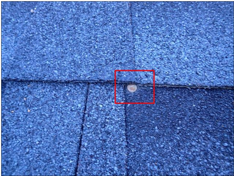
C. Item 5(Picture) Multiple nail locations
