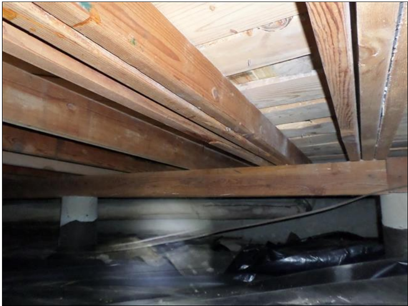
A. Item 2(Picture) No floor insulation
